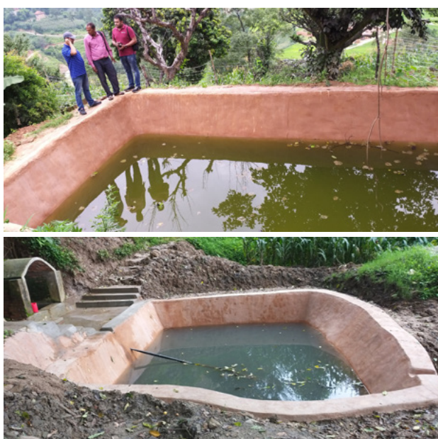
Plate 13. Soil-cement ponds constructed at Kavre
